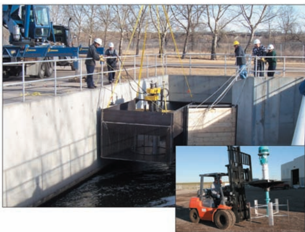
First 5kW prototype VAHT water current turbine installation at Bonnybrook Wastewater Treatment Plant in Calgary (Inset): Fully assembled VAHT generating system
